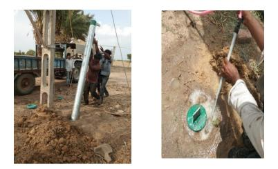
**Present System:** Presently, the earthing practice followed by all DISCOMs is generally to install the salt charcoal type earthing system. The earth pit is erected with the augur or manually. The earth pit is filled with layer of salt and charcoal. As the earth electrode coil made of GI wire is used or GI plate is used. In some urban installations, maintenance free earthings are used but that is also having very limited application due to quite high cost.
